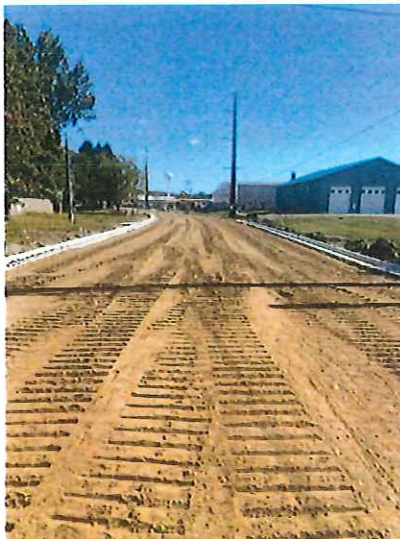
Left: 1st Street SE looking east from Dolphin Avenue. Graded aggregate base being prepared for bituminous paving. Above: Upcoming bituminous paving work schedule to begin on October 10th
